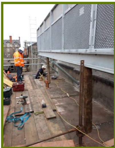
DC474 - St Georges Ave Signal Platform Installation
