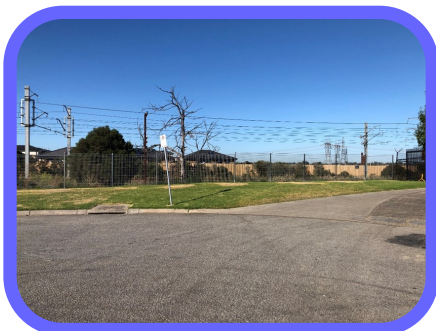
Completed works at Len Thomas Plane, Narre Warren, VIC.
