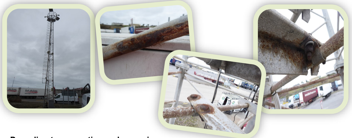
Descaling tower section and preparing for painting.
