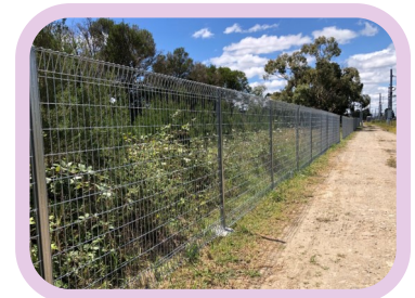
Completed works at Officer Station
