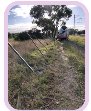
Progress works at Officer Station
