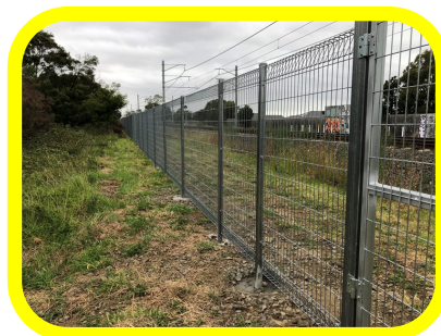
Completed works at Cardinia, VIC
