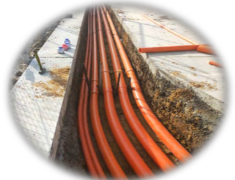
Conduit run from SS to property boundary
