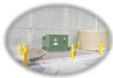
Bollards installed, stone added & concrete upstand poured
