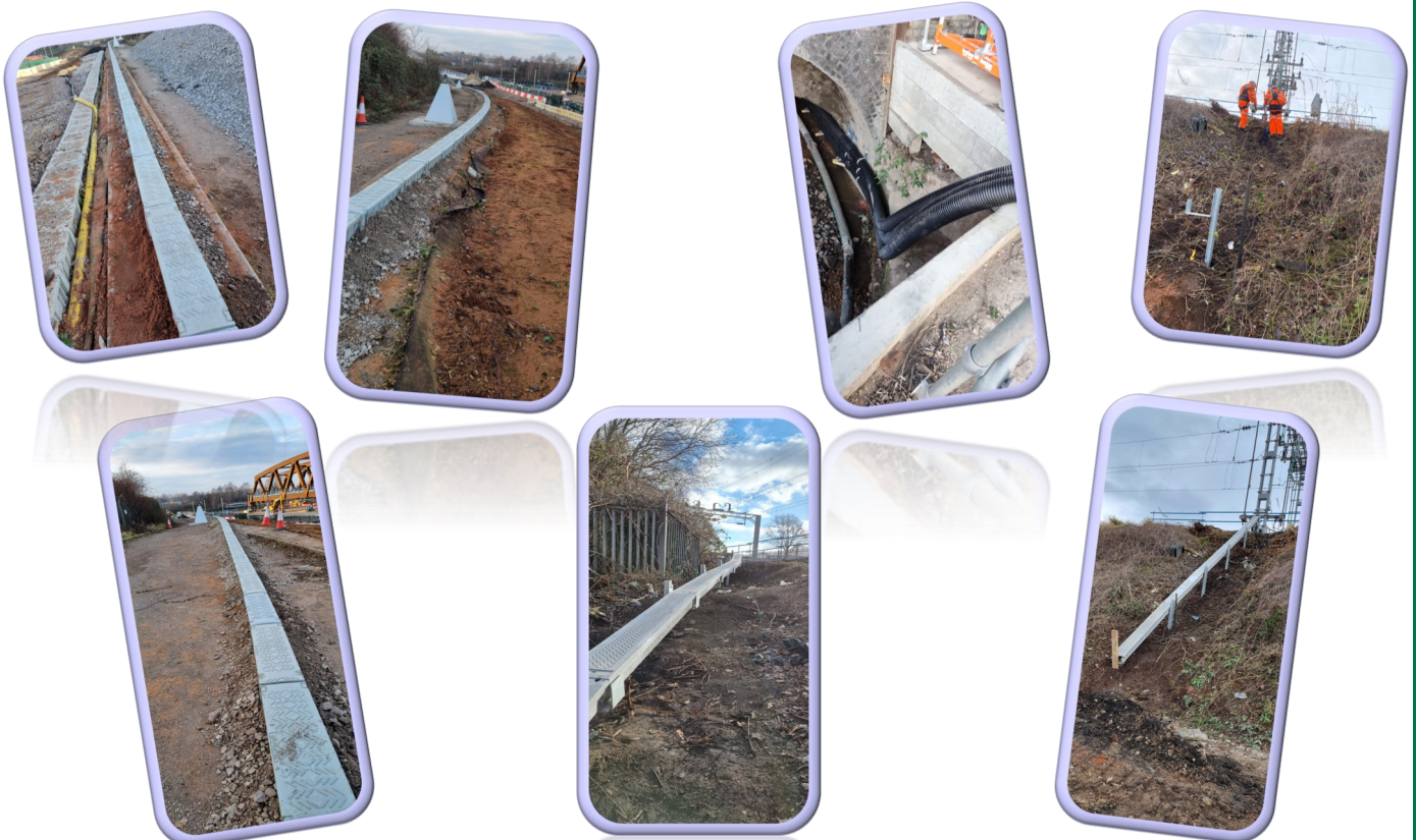
The images show the route work installation for the HV OLE diversion with works progressing nicely
