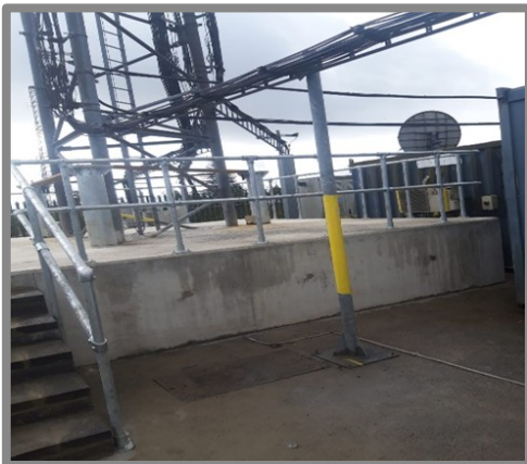
New Plinth Built Over Existing Base
