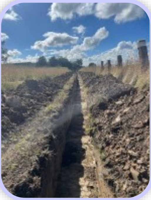
Trench open, ready for conduits installation
