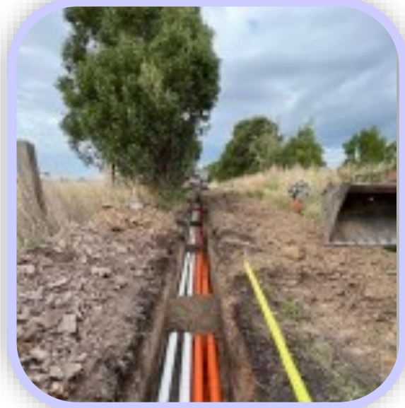
Conduits installed as per design
