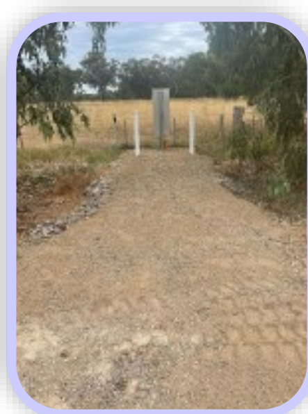
Completed meter post
