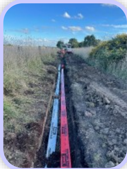
Traceable Marker Tape installed & backfill & compaction of trench
