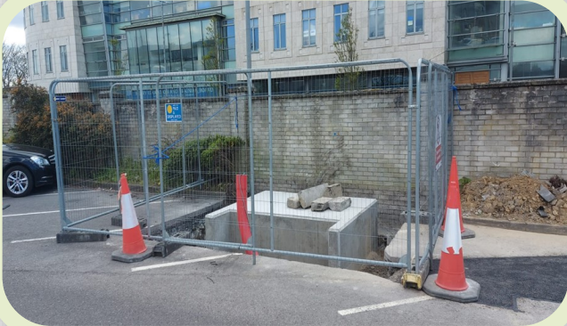
ESBN substation base constructed in Tralee
