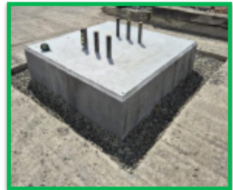
In-situ foundation boxes installed to support the new terminating columns
