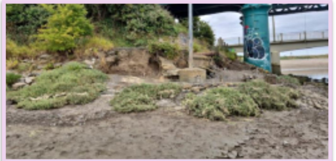
BEFORE Washed Out Embankment at the Northern Abutment
