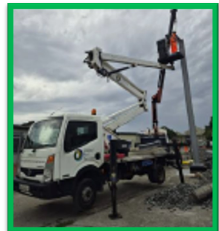
Working at heights to install the columns
