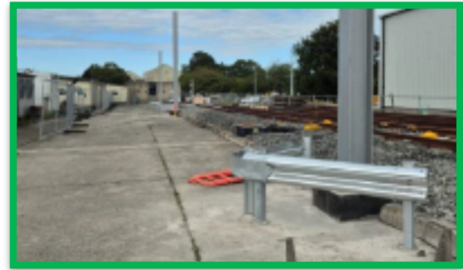
Armco rails installed to protect the newly placed columns
