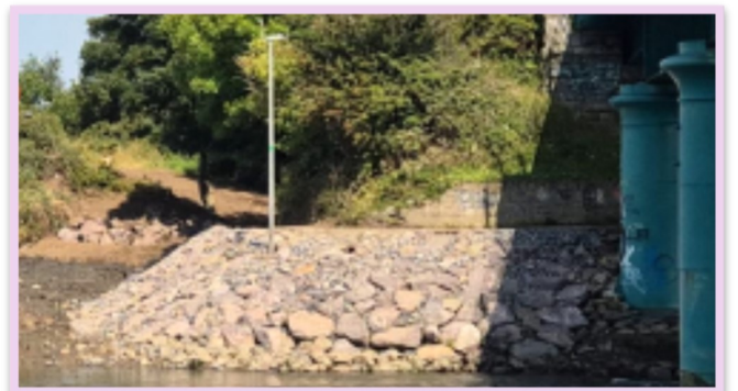
AFTER Newly Installed Rock Armour at the Northern Abutment
