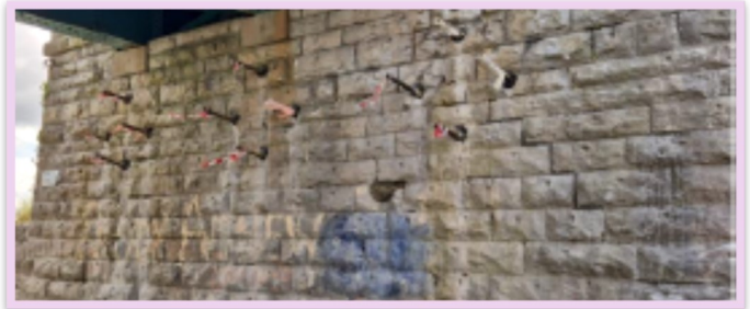
Southern Abutment Masonry Repairs
