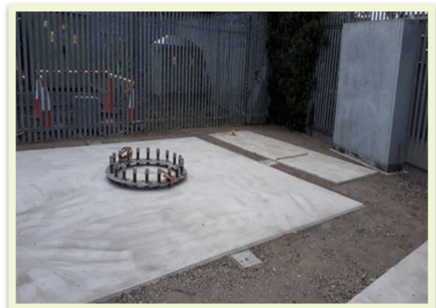
Plinth ready for Monopole Installation
