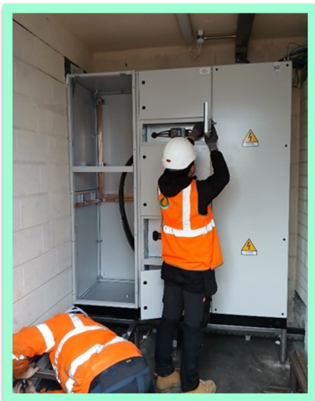
Delivery & Installation of Low Voltage Distribution Board
