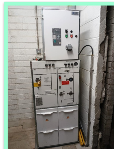
MV Switch Installed & Operating
