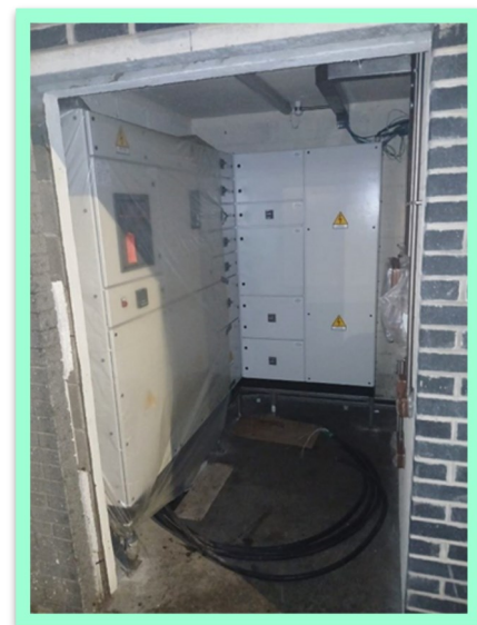
Delivery & Installation of Low Voltage Distribution Board
