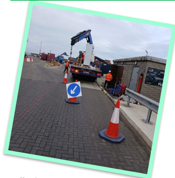
Delivery & Installation of Low Voltage Distribution Board
